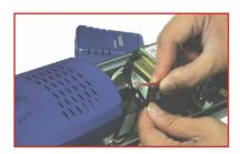
**12.** Place the yellow wire connector over the assembly in step 11, and twist the wire connector clockwise to secure the contact between the wired pair.
